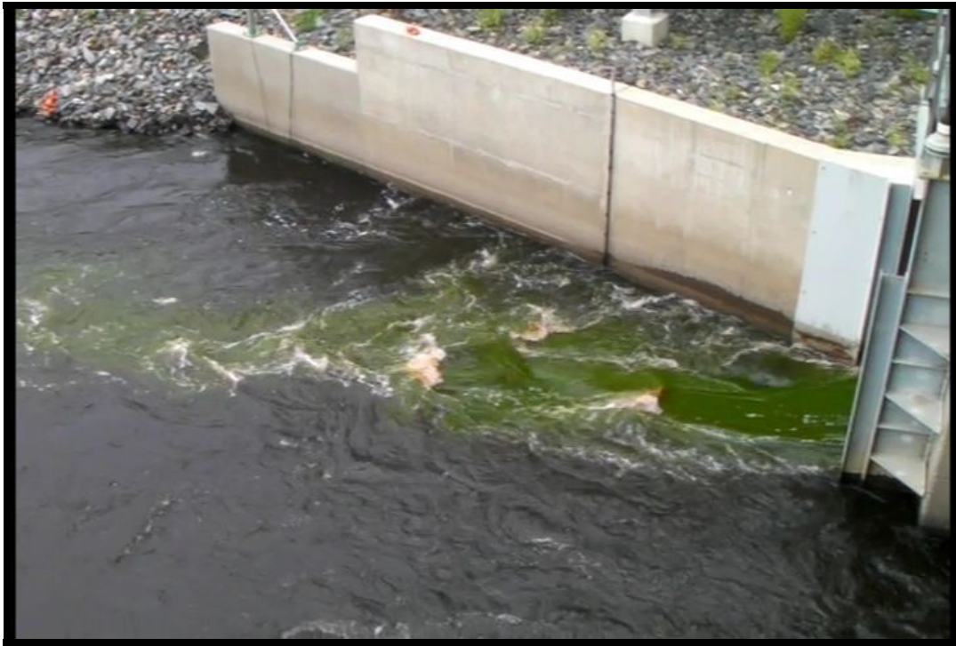
Photo 2: Between 0 and 75' downstream of fishway entrance area.
