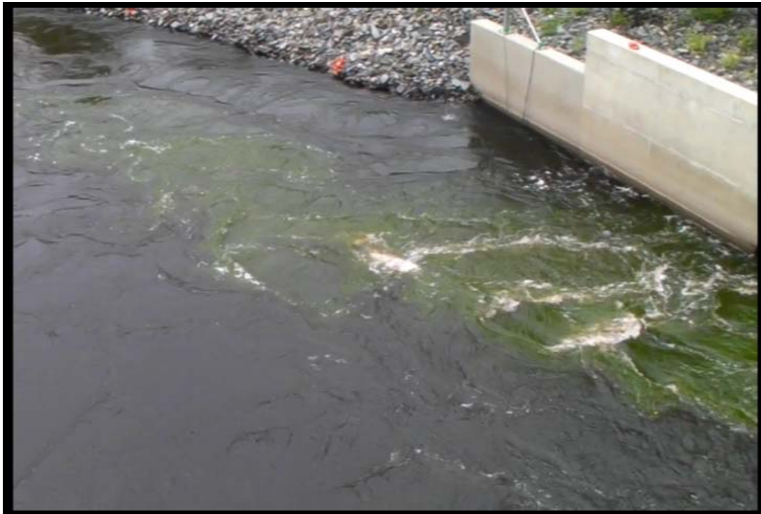
Photo 3: Between approximately 25' and 100' downstream of fishway entrance area.
