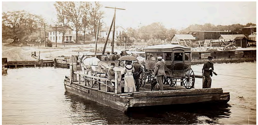
Cable crossing type ferry, Pentwater, MI
