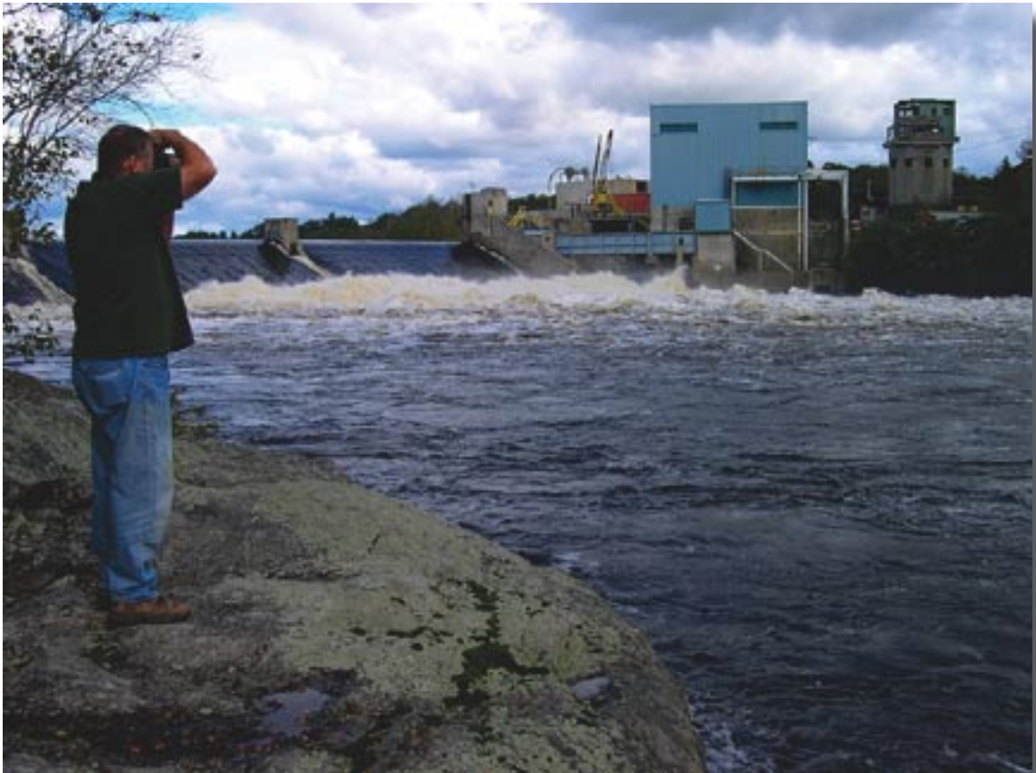
Expert witness Randy Bailey photographs Pejepscot dam's upstream approach on the Andro
