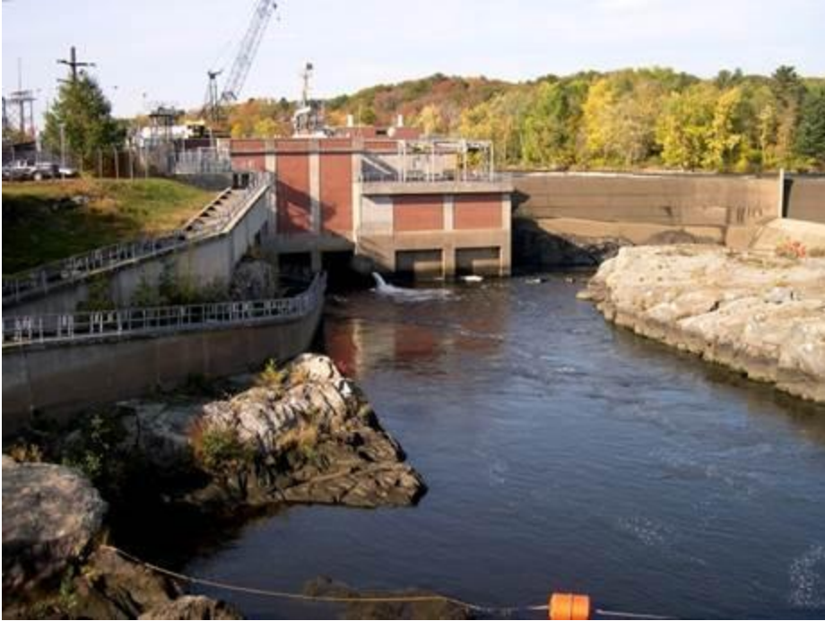
Brookfield Energy's Androscoggin River dam between Brunswick and Topsham. CREDIT ED FRIEDMAN, FRIENDS OF MERRYMEETING BAY
